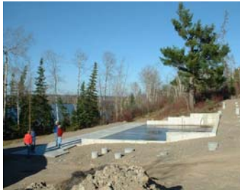
Foundation slab for the Baypost
