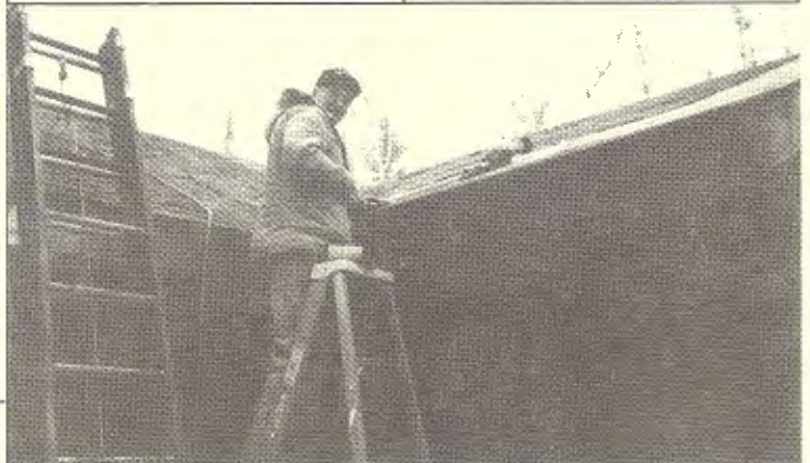
Dick Hall fits new shingles on lodge roof and closeup near fireplace shows new cedar fascia around the new insulated roof addition.
